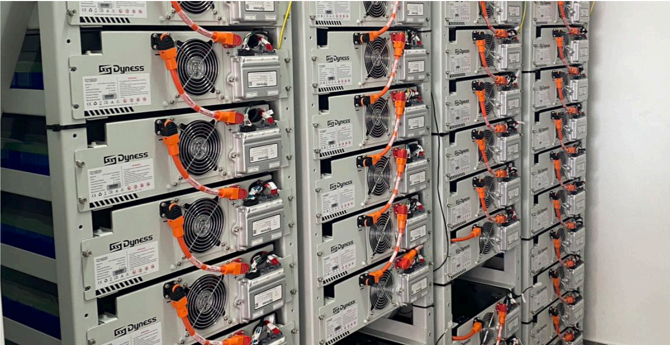
• Lebanon PowerRack HV4F Capacity: 215kWh Self Generation and Consumption
